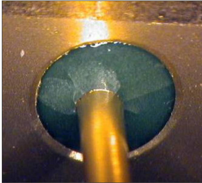
Figure 8 – Leak failure from glass feedthrough crack
